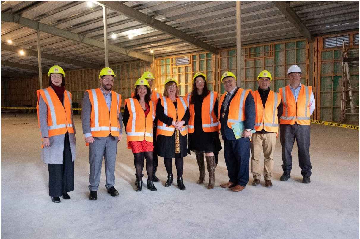
Inside the new MSL Building being constructed at Gracefield, Lower Hutt
